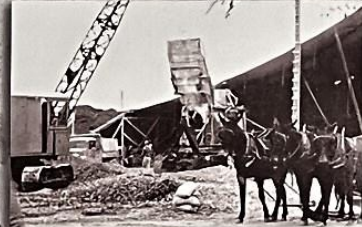
A crane with clamshell bucket for excavation, a dump truck and a team of mules – all manner of "horsepower" was used to build the Monument.
