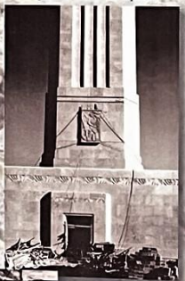
Finishing touches – a stone frieze panel is lifted into place.
