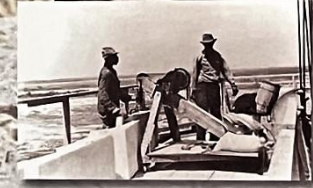
Using a small lift, two men maneuver an 8,000-lb. block of limestone into position.
