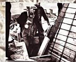
A mock-up of the star was built on the ground to test the assembly of a star that would have five points from any viewing angle.
