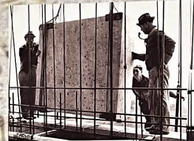
Hoisting a large stone in place on the Museum. Note the microphone for directing the crane operator.
